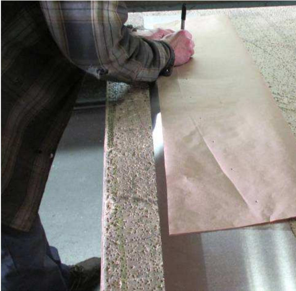
Wait to drill the holes. It is best to drill the holes using a hole-finder.
