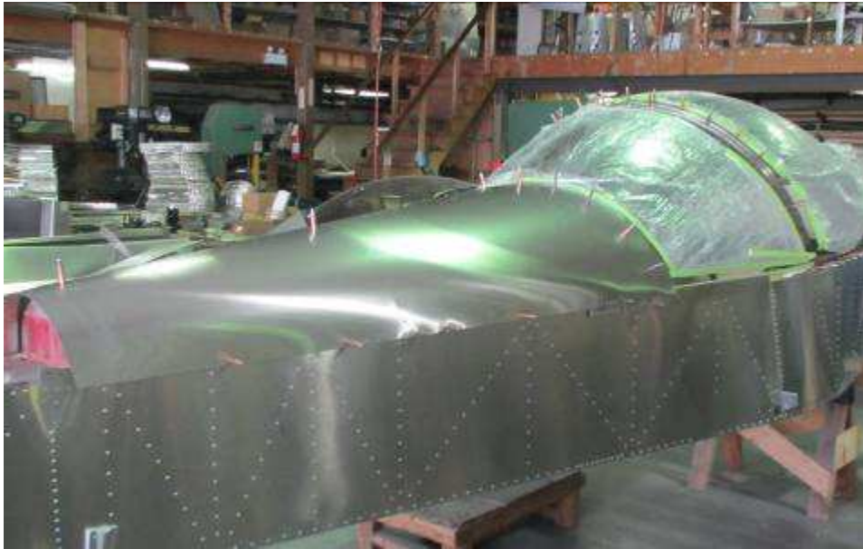
Cleco the rear skin to the fuselage and bulkhead
