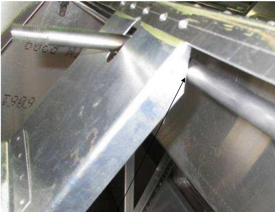
Snip off the top corners on the side flange of the channel.
