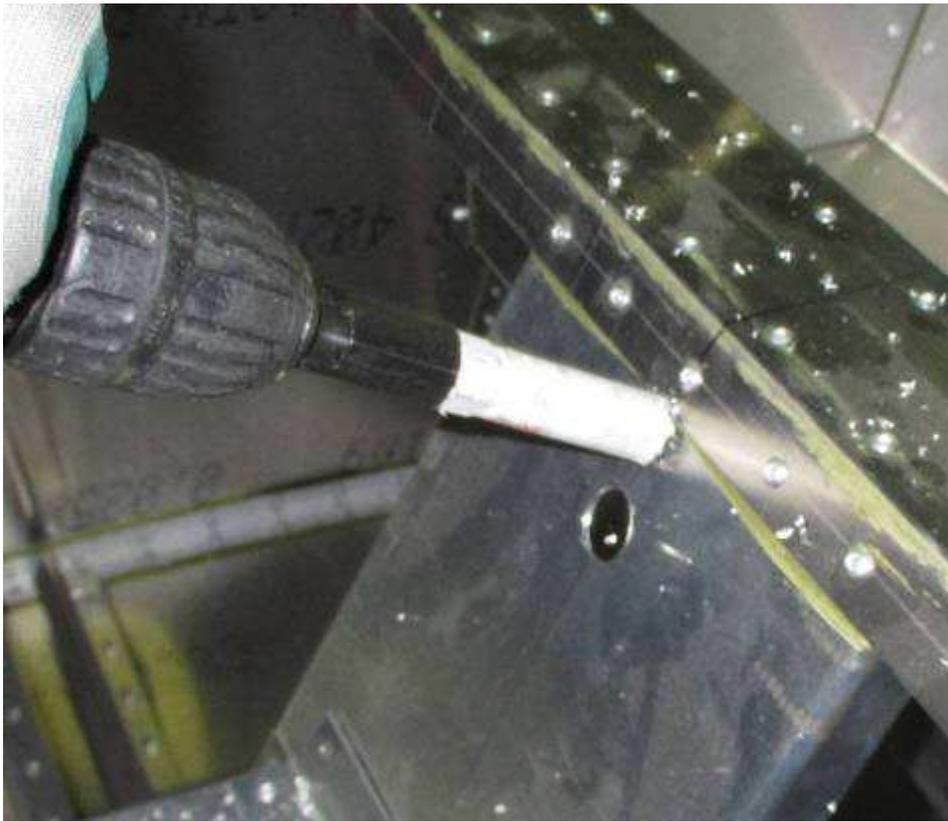
Open up with a 3/4" hole saw or uni-bit
