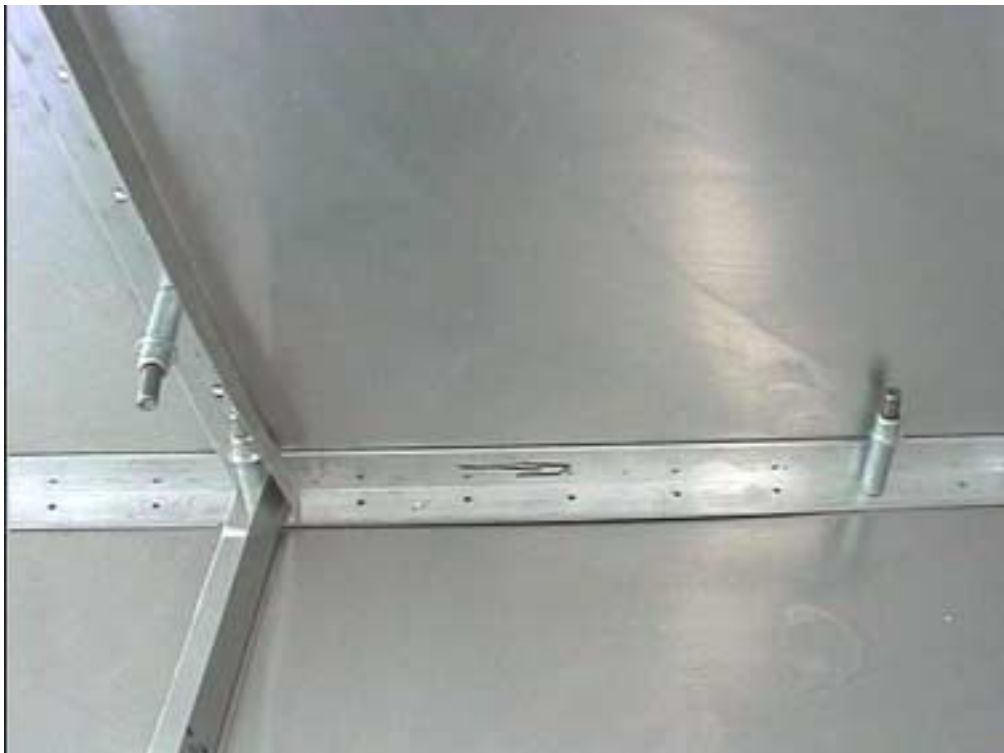
Note: There is no gusset or rivet in the overlapping flange of the vertical and horizontal L angles.
