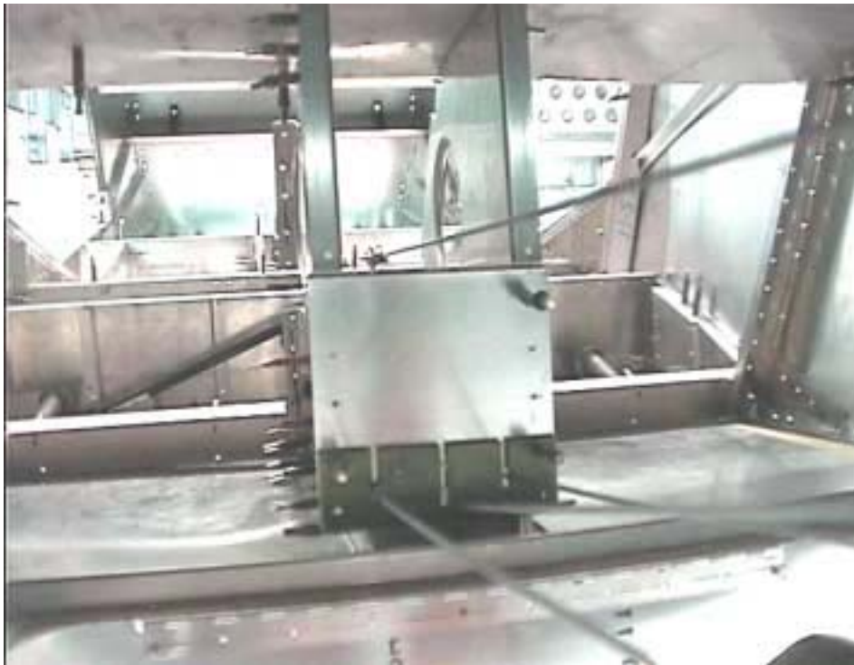
Looking at the rudder and elevator cables through the a back side of the Horizontal Tail Bearing Support Channel 8C1-2
