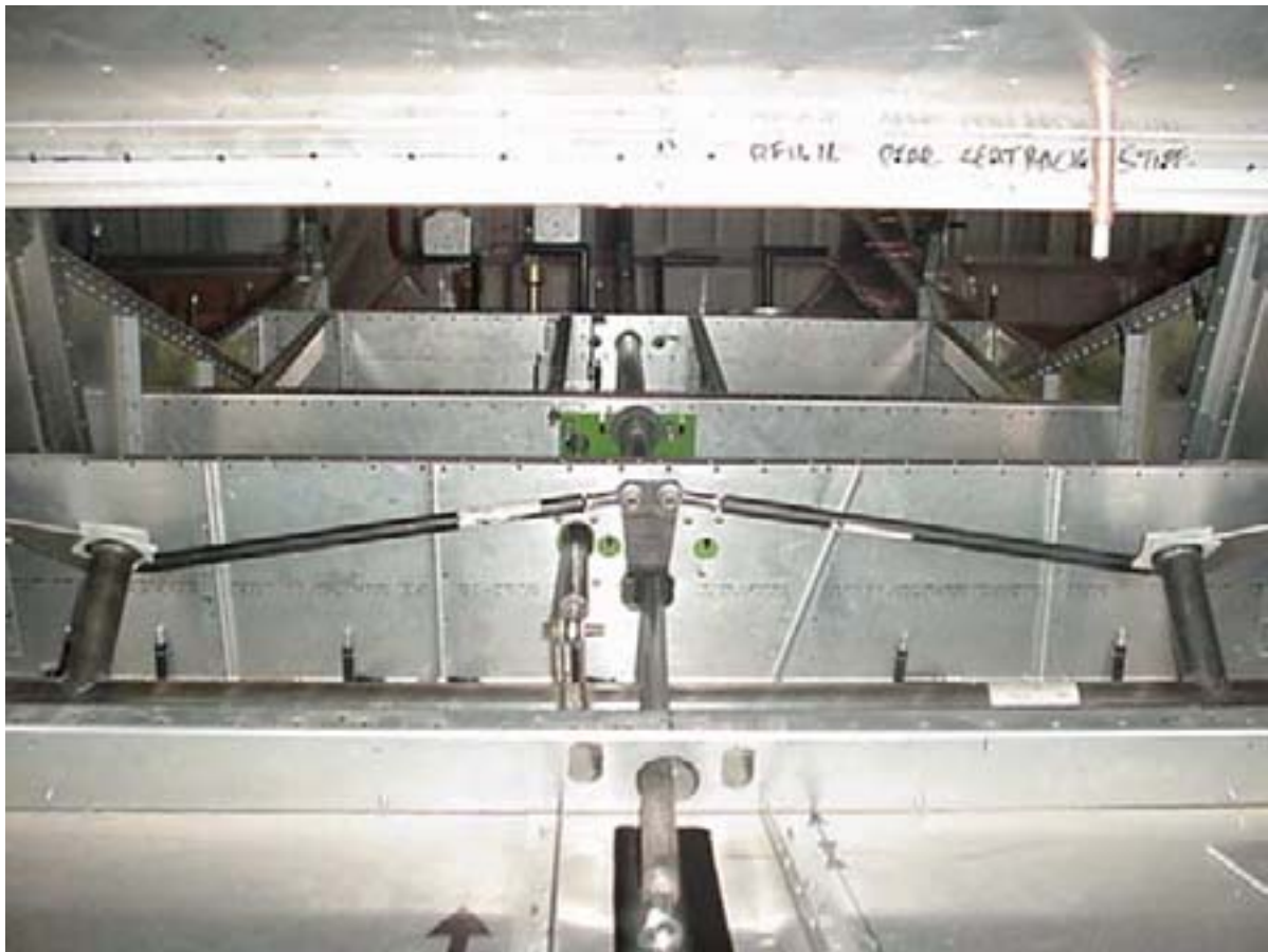
Rear seat back and seat bottom removed. Photo taken from the rear fuselage access hole looking forwards at the Horizontal Control Rods 8C9-1
