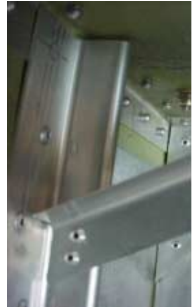
2 RIVETS A4 L angle into 7F7-5
