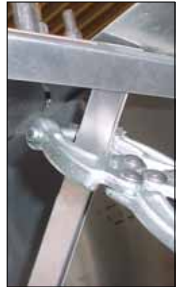
L angle overlaps behind the top and bottom angles 7V8-2 and 7V8-3.
