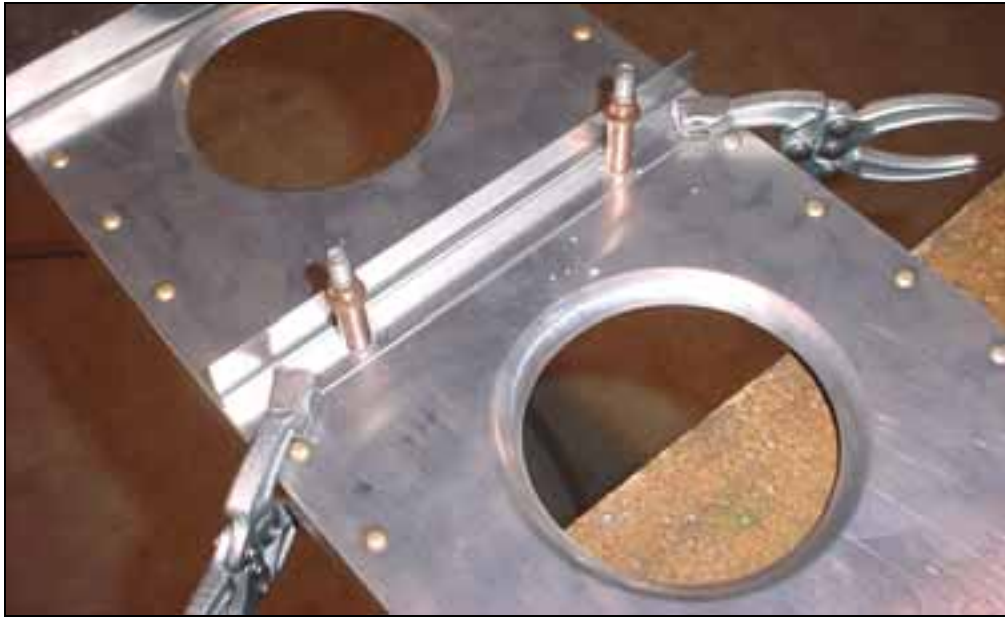
Drill and cleco with #30 drill.
